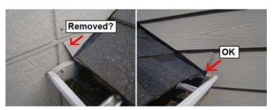
(C) The right side dormer flashing nail wasn't sealed with mastic like the others and it is rusted. Recommend correcting this condition(s).
