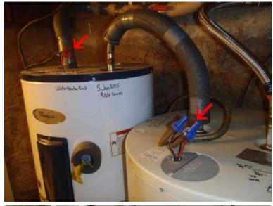
(S) The electric clamp is missing on the laundry room water heater. These conditions are a safety hazard. Recommend correcting these condition(s).
